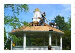
Old shingles were removed, along with the railing around the cupola, and then the rotted wood was replaced. A waterproof liner that was supposed to seal the flat part of the rood from water had failed, so it was replaced with a new state-of-the-art liner. Then new shingles were installed.
